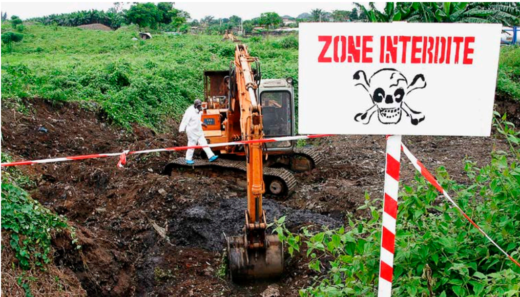
Clean-up work at one of the contaminated sites
